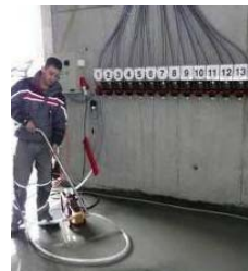
Filling station AFS
